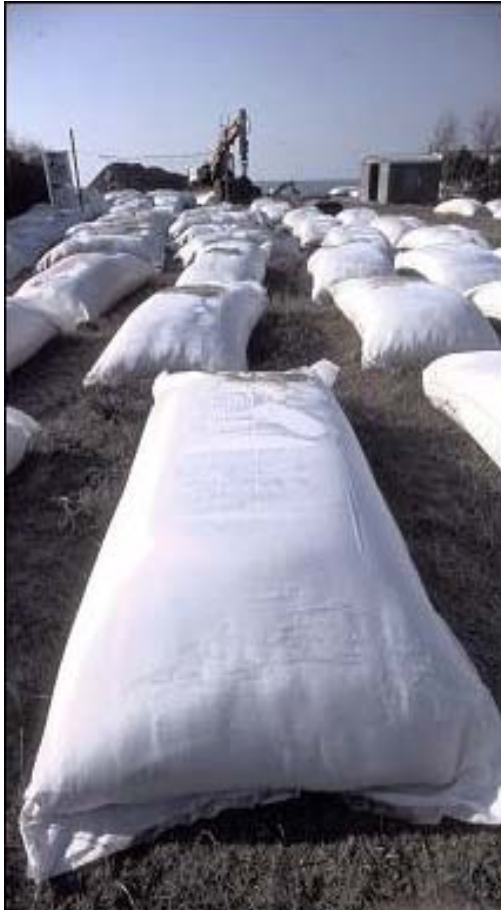
Figs. 13, 14 & 15: Sand bags and construction works of experimental submerged groins.
