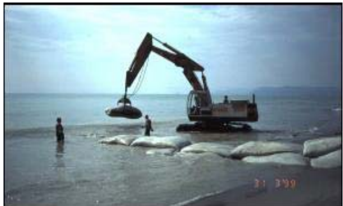
Figs. 13, 14 & 15: Sand bags and construction works of experimental submerged groins.
